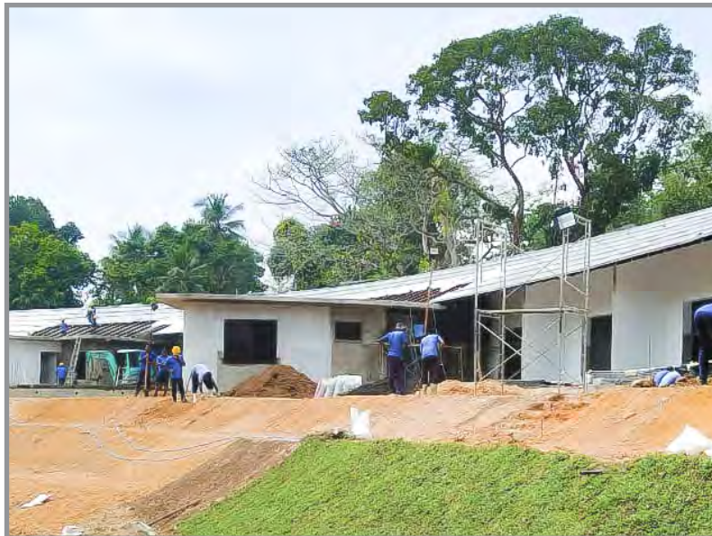
Construction of "Transit Home" in Galle
